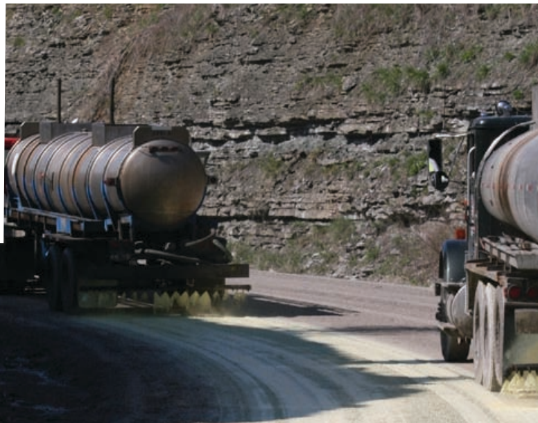
Haul road is spray treated to prevent coal dust.
